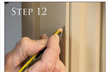
After marking the top and bottom of the latch open the door and continue the marks around the door frame to get final resting position of your latch.
