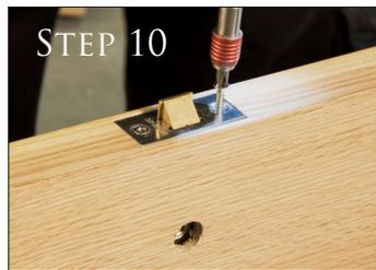
With the faceplate in position drill pilot holes and fix the latch in place using the screws provided.
