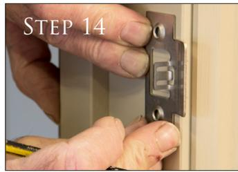
After step 13 hold up the receiver plate to your door frame so it is centralised with your latch lines on the wood and the door line on the back of your receiver. This gives excellent position for fitting the plate.
