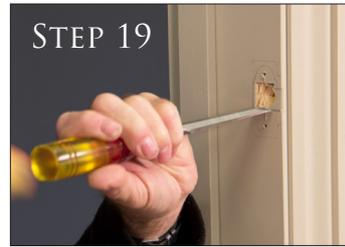
Chisel out the main square area deep enough for the tidy to fit snugly into and proceed to carefully chisel out the outline previously drawn for the receiver plate to sit flush with the surface of your frame.
