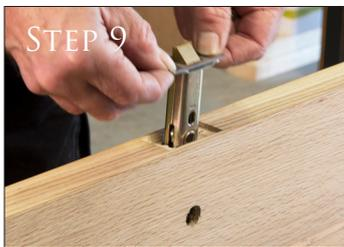
Now is the time to insert the latch with its faceplate into the edge of the door and make sure everything fits flush.
