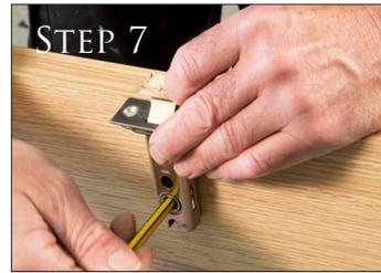
The next step is to get position for the spindle which passes through the door latch and connects your two handles together.
