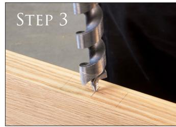
Using your pencil cross which should be centred in the outline of the latch faceplate drill into the door edge using an auger drill bit. The size of bit depends on the size of the latch casing so make sure it is big enough so that the latch will slide into the door easily. It is worth doing this drilling now as when you start chiselling all pencil marks will be removed.
