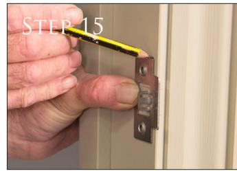
Hold the plate firmly in position and with a pencil draw around the outer part of the receiver, the two fixing holes and the hole (for the latch to fit into).
