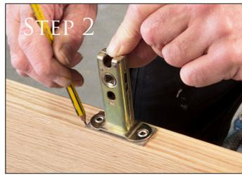
With the square face plate held onto the latch position on your pencil mark and centrally on the edge of the door.
