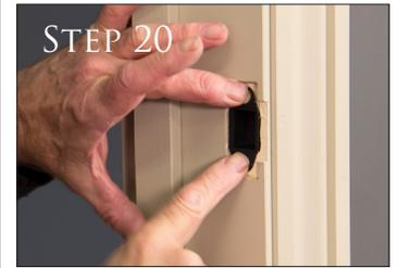
Position the latch tidy in place to confirm it all fits well and place the receiver over the top of this.
