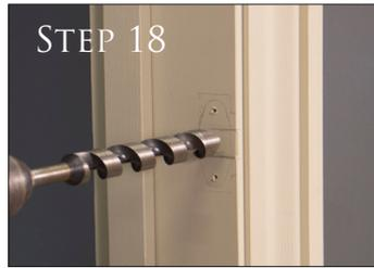
Using your guide hole in the centre drill out using an auger bit enough space for the black plastic latch tidy to fit comfortably into.
