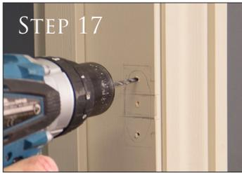
With all your marks made it is always a good idea to drill any holes need before you begin any chisel work as all marks will be removed.
