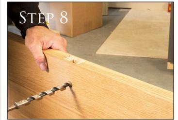
Using the mark you have just made through the spindle hole of the latch it is time to drill all the way through the door. This allows the spindle to pass from one handle through the door, operate the latch and connect the handle on the other side.
