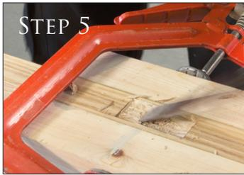
Once the outline has been made begin to carefully chisel out enough of the door edge so that the latch and faceplate will sit flush with the surface.
