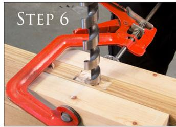
Using the pre-drilled hole you may want to re-drill using the same auger bit just to make sure the latch casing will fit properly and to the right depth also.
