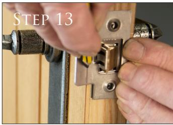
A good trick here is to hold up the receiver plate to the position of the faceplate on the latch and mark on the reverse of receiver where the edge of the door sits.
