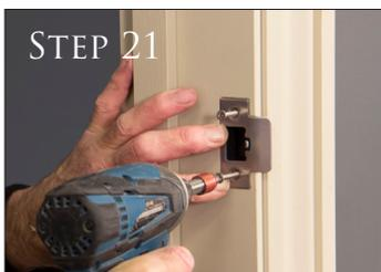
Using your pilot hole from before fix both the tidy and the receiver plate in place using the fixing screws provided.
