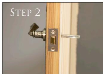
Firstly you will need to fit the spindle (square metal bar) to the back of one of your handles. This spindle will then pass through the hole in your door which when turned will operate the latch (or lock) mechanism already fitted in your door.
