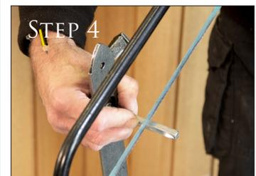
Once you have measured the amount of spindle that needs to be removed mark it on the end of the shaft and using a decent hacksaw remove that portion.
